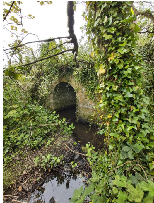
B. Crossing point between the Normansgrove Stream and the L1010 route
