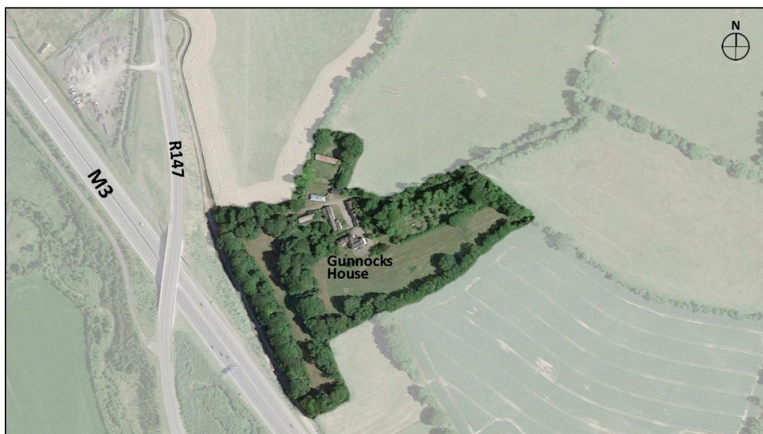
Figure 11.5 Gunnocks House and woodlands adjacent to R147/M3 overbridge
